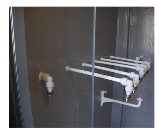
Holes made through the structure were filled with a bathroom grade sealant.
